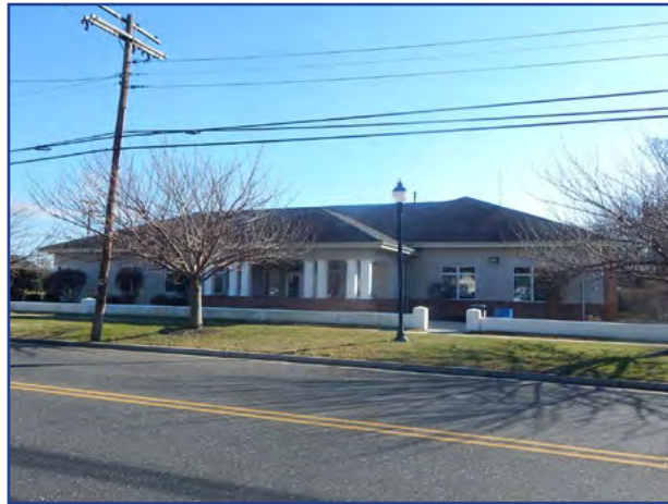
Woodbine Municipal Building
