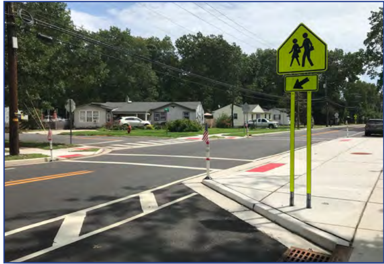
Traffic calming measures to increase pedestrian safety at the recently renovated intersection of Webster Street and Madison Avenue at the entrance to the Woodbine Community School
