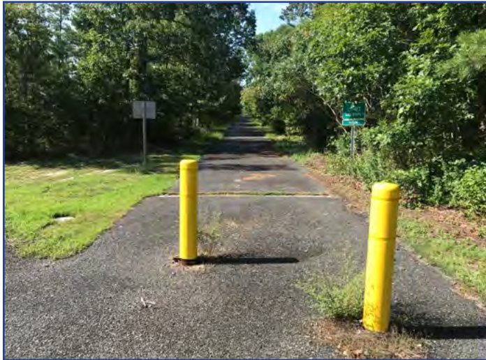
Entrance to the Airport Spur Bicycle Path
