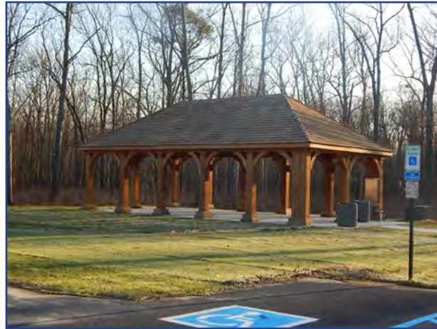
Pavilion completed during Phase I of Eco-Park Construction
